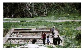
It's an odd building for China: high passive solar gain, which means it is a heat sink. It has walls that are two layers of brick on one side and on the other, with about 1ft. of volcanic ash in between. Double paned windows. It was designed in Boulder Colorado by Adrian Sopher and Paul Kloppenburg. It was a tough project to do because the blueprints had to be translated
